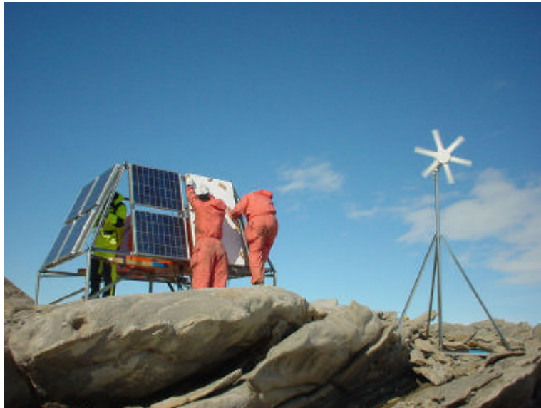
Fig.3 GPS remote base station at Langhovde. GPS antenna is mounted on a nearby separate pillar.
